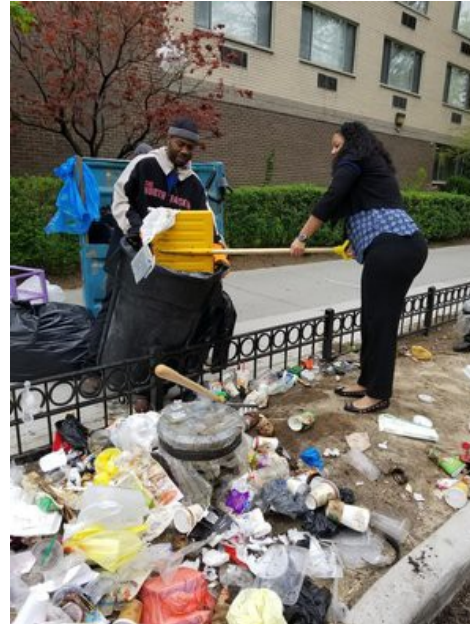
Bioswale filled with trash - Queens Examiner
