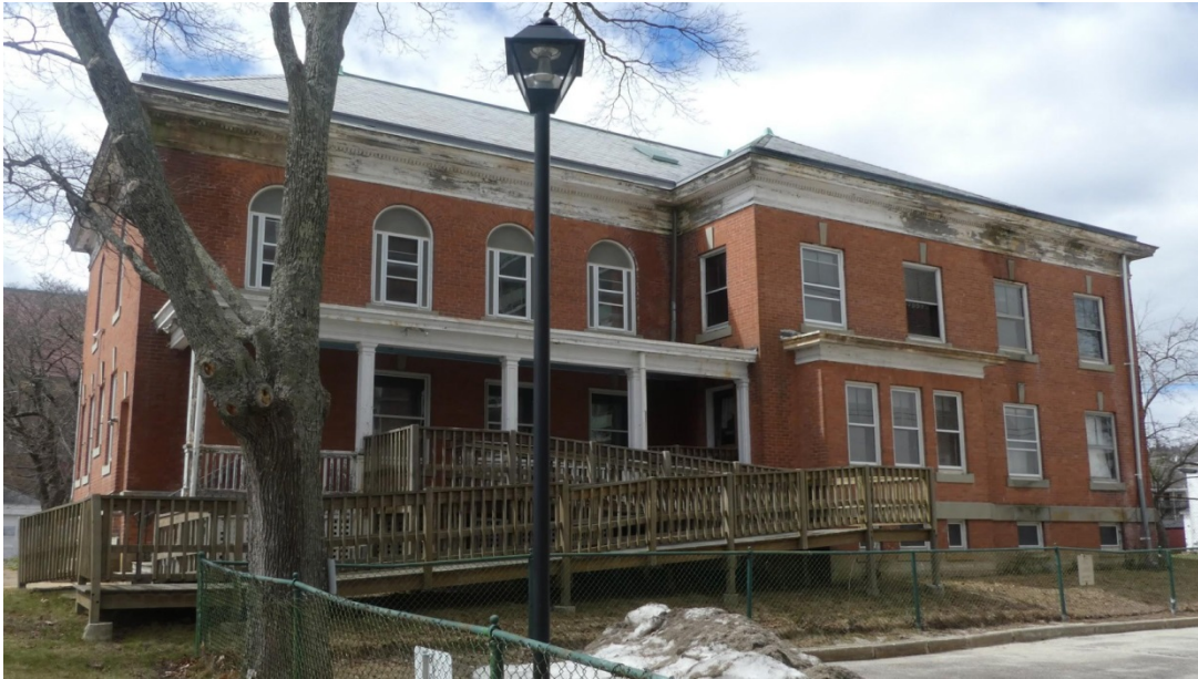
Figure 6-2. The east side of the convent. (Photo by Josee Uwayezu)
