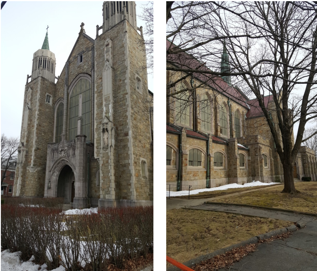
Figure 2-1. Exterior of the Sacred Heart Church building.
