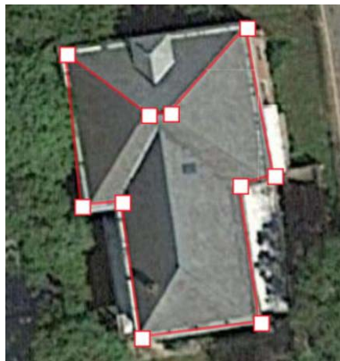
Figure 6-15. Aerial view of the convent roof. (Image from Google Earth)
