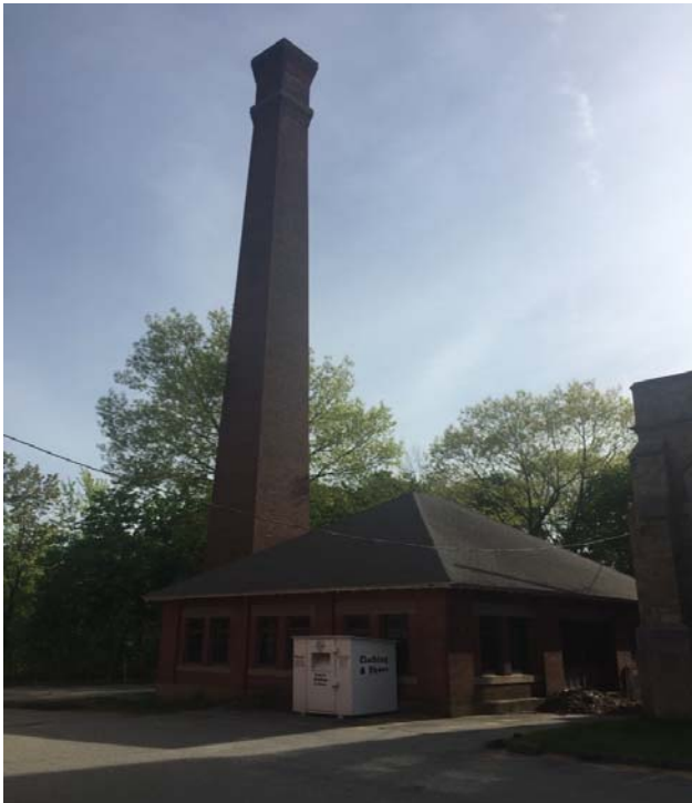
Figure 3-1. Power plant – East facing view.
