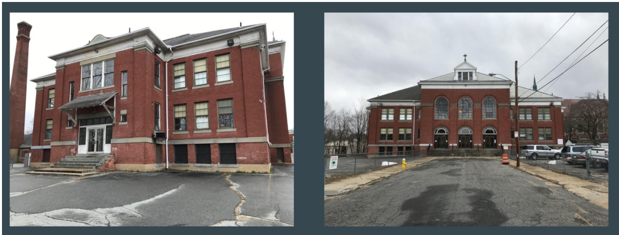
Figure 7-1. Typical sights on the Sacred Heart Church campus with paved driveways and parking areas.
