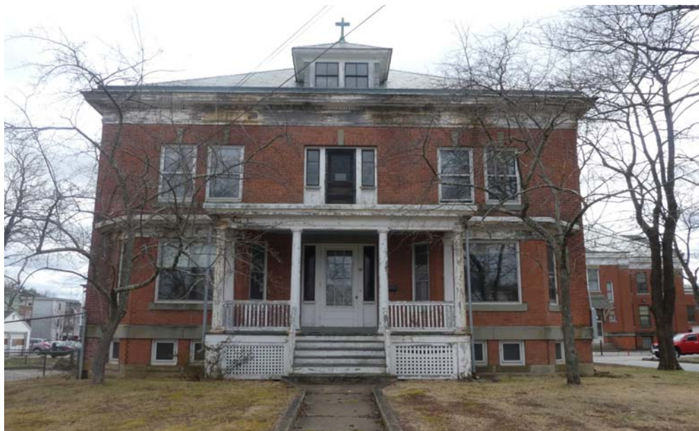
Figure 6-1. Northern façade of the convent. Notable architectural features of the convent are the keys over the windows and the box cornice at the roof. (Photo by Josee Uwayezu)
