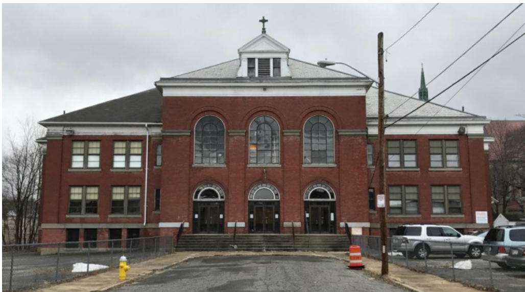
Figure 4-1. The façade of the school building, facing east.
