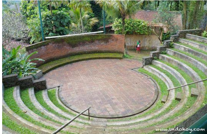
Figure 7-4. Example of a water collection amphitheater, which serves the dual purpose of impounding water after rainstorms and outdoor performance arena in dry periods 122 .
