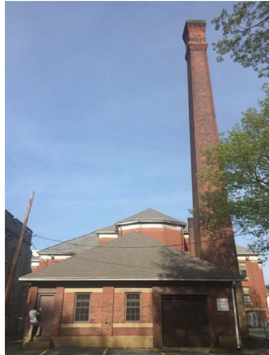
Figure 3-2. Power plant. West facing view, with loading dock. The church building is seen in the rear.
